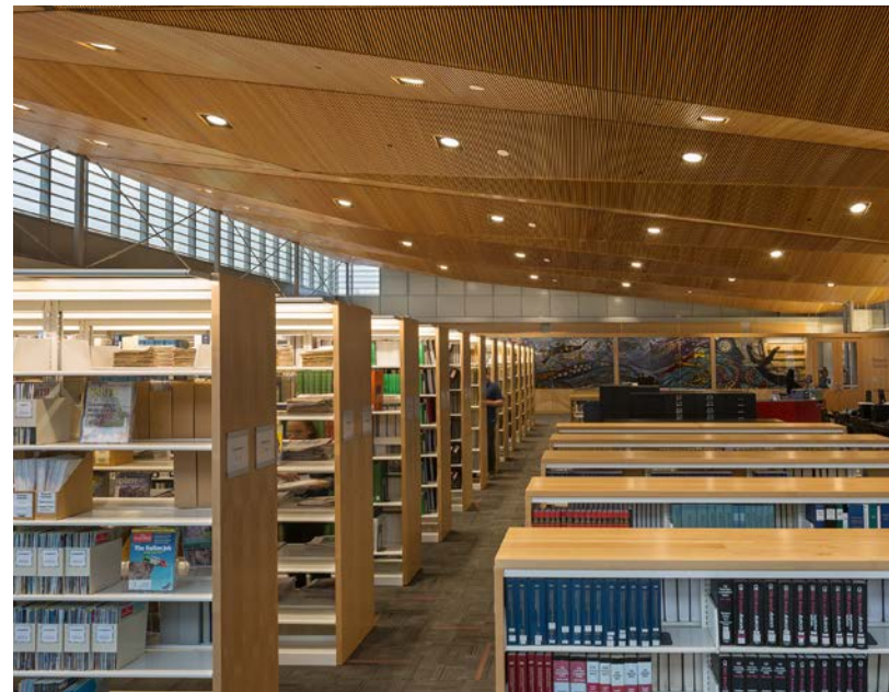
In the library, the wood grille ceiling's compound, pie-shaped sections flow from a height of 22' down to 16'.
