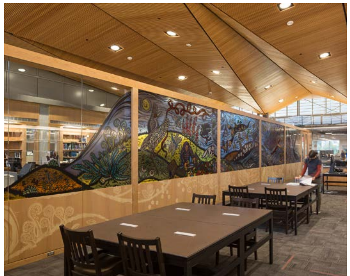
The state library, archives and museum features 21,250 sq ft. of solid Western Hemlock, wood grille ceilings in its lobby, library, and reading room.
